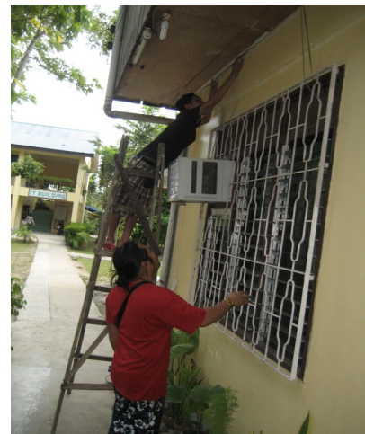
September 9, 2014 Installation of CCTV on designated areas for added security.
