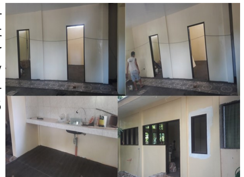
New homotel extension under construction
